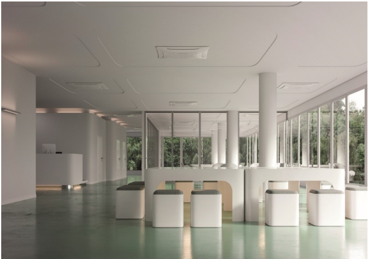
Picture of the installed SK-ECM Fan Coil
