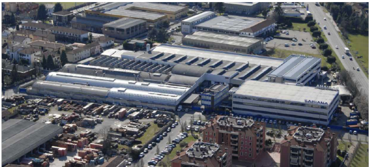
Aerial view of Sabiana headquarter
